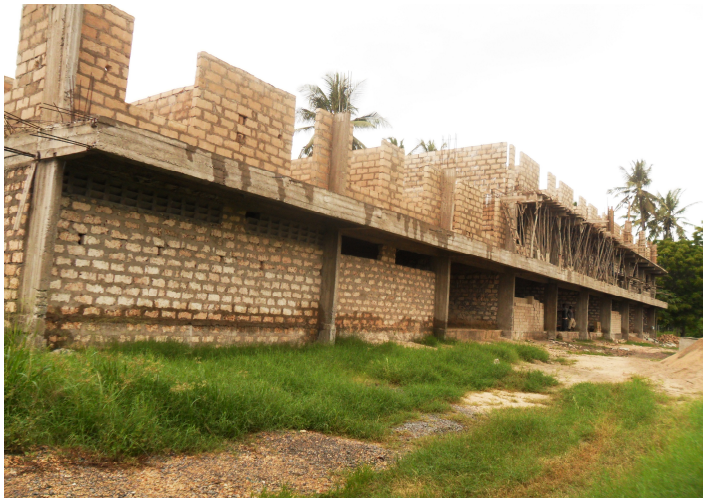
Under construction – the proposed flats for the Ustadhs of our institution
