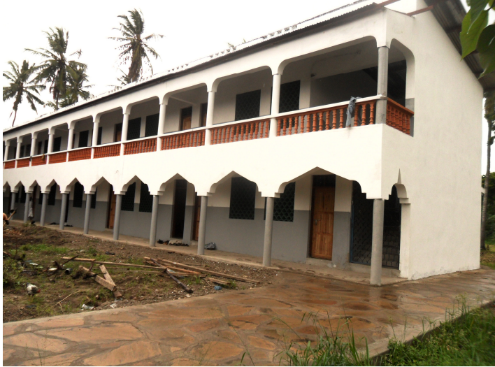
The new addition – The newly constructed hostel
